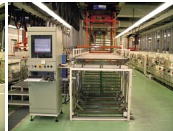
Automatic rack plating line in the Montblanc plating shop
