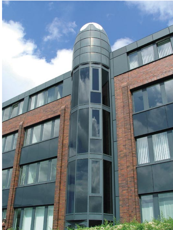
Montblanc in Hamburg: the administrative building with stylised fountain pen cap as a stairwell.
